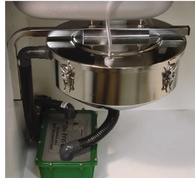
Amalgam separators (pictured) can be easily attached to dental chairs to capture waste mercury, keeping it out of waterways.
